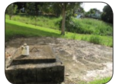
Keep septic tanks sealed.
